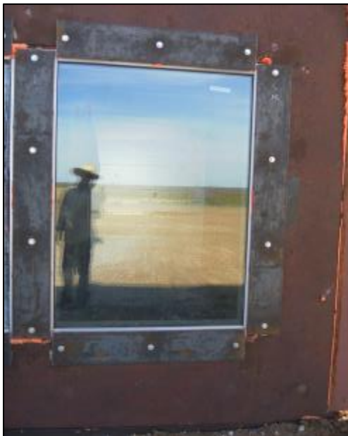
Photo No 215 Post-test, Exterior Specimen 28
