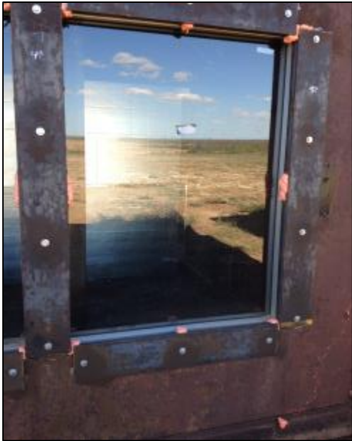
Photo No 66 Pre-test, Exterior Specimen 8
