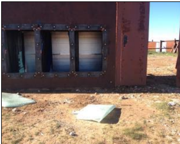
Photo No 40 Post-test, Exterior Specimen 4
