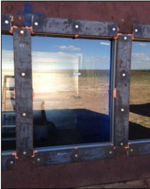
Photo No 25 Pre-test, Exterior Specimen 3
