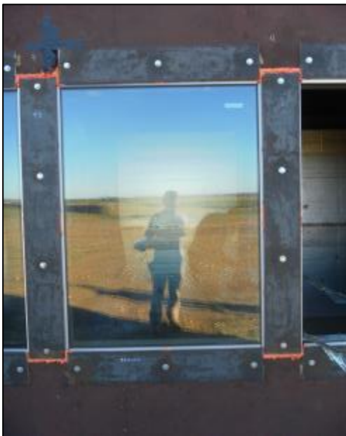
Photo No 144 Post-test, Exterior Specimen 19
