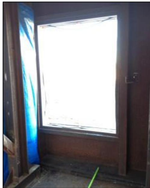
Photo No 4 Post-test, Exterior Specimen 1
