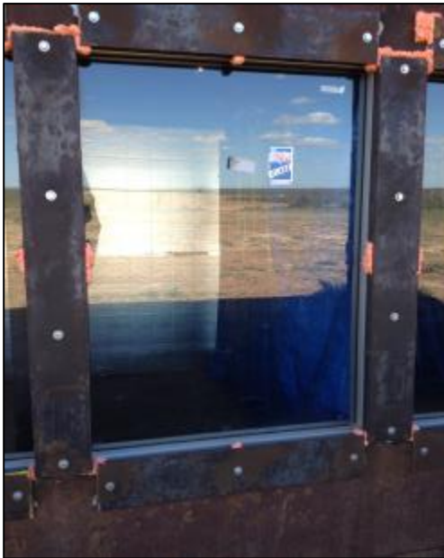
Photo No 57 Pre-test, Exterior Specimen 6
