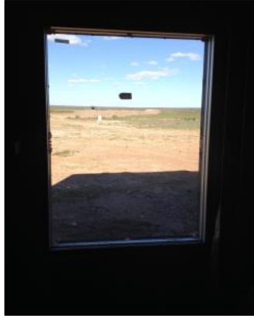
Photo No 39 Pre-test, Interior Specimen 4
