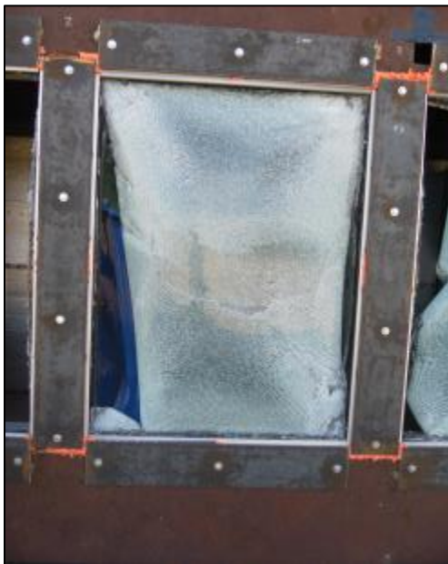
Photo No 202 Post-test, Exterior Specimen 26
