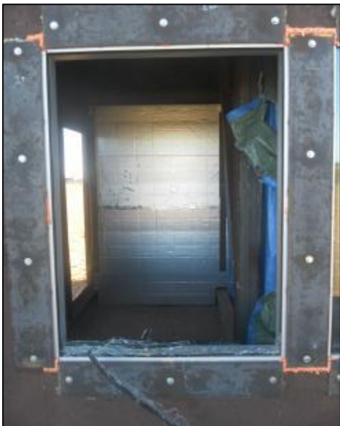
Photo No 126 Post-test, Exterior Specimen 17
