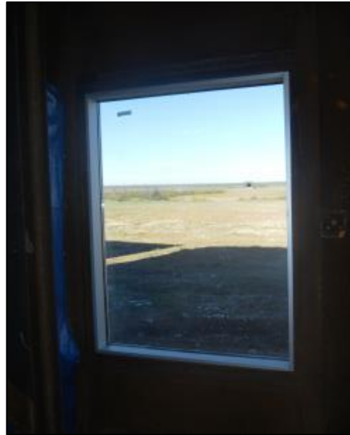
Photo No 154 Pre-test, Interior Specimen 21
