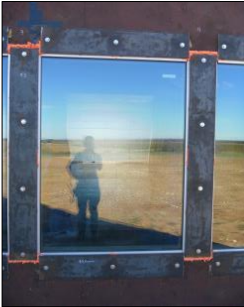
Photo No 142 Pre-test, Exterior Specimen 19
