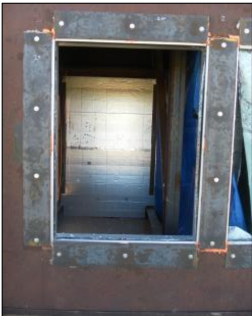
Photo No 197 Post-test, Exterior Specimen 25
