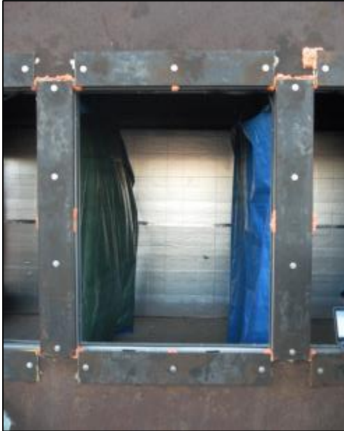
Photo No 108 Post-test, Exterior Specimen 14
